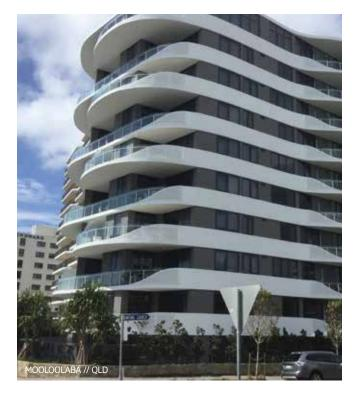
Cemintel Commercial RendaLine<sup>®</sup> is a complete external cladding system that incorporates all the advantages of lightweight construction with a flush-jointed, texture coat finish.
