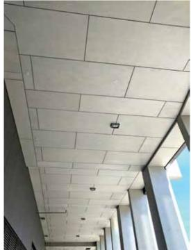
Barestone<sup>™</sup> provides significant design flexibility. If used internally or externally as a wall cladding, the look can continue through to ceilings eaves and soffits.
