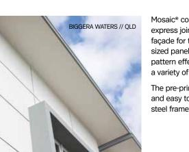
Mosaic<sup>®</sup> combines a modern, geometric express joint aesthetic making it the ideal façade for the modern home. Multiple sized panels can be arranged to form a pattern effect either using block colour or a variety of tones using a painted finish.
