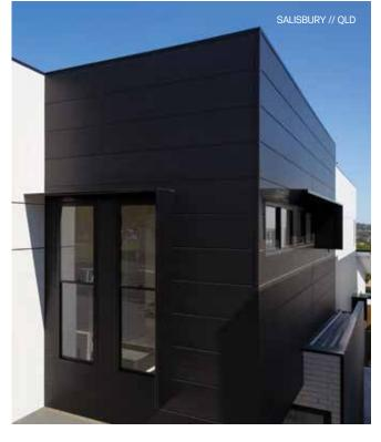
The 300mm wide Cemintel Aspect Cladding<sup>®</sup> panel displays a single and visible 16mm wide groove, providing easy coverage for an attractive façade.
