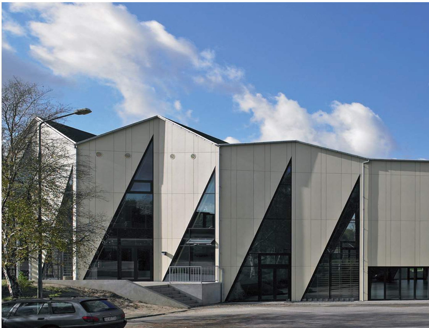
DENMARK Sports Hall Kibaek Krydsfelt, Kibaek
