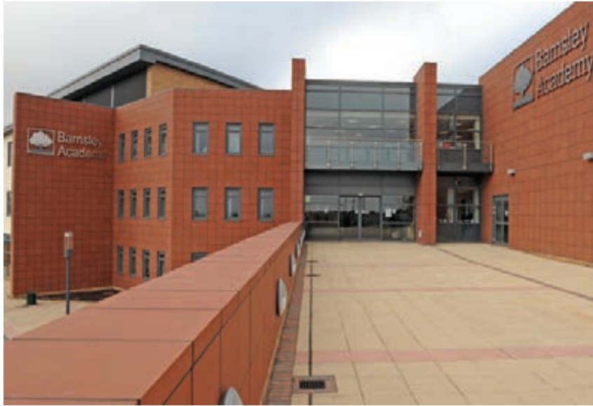
Barnsley Academy Rainspan with Terracotta Tile
